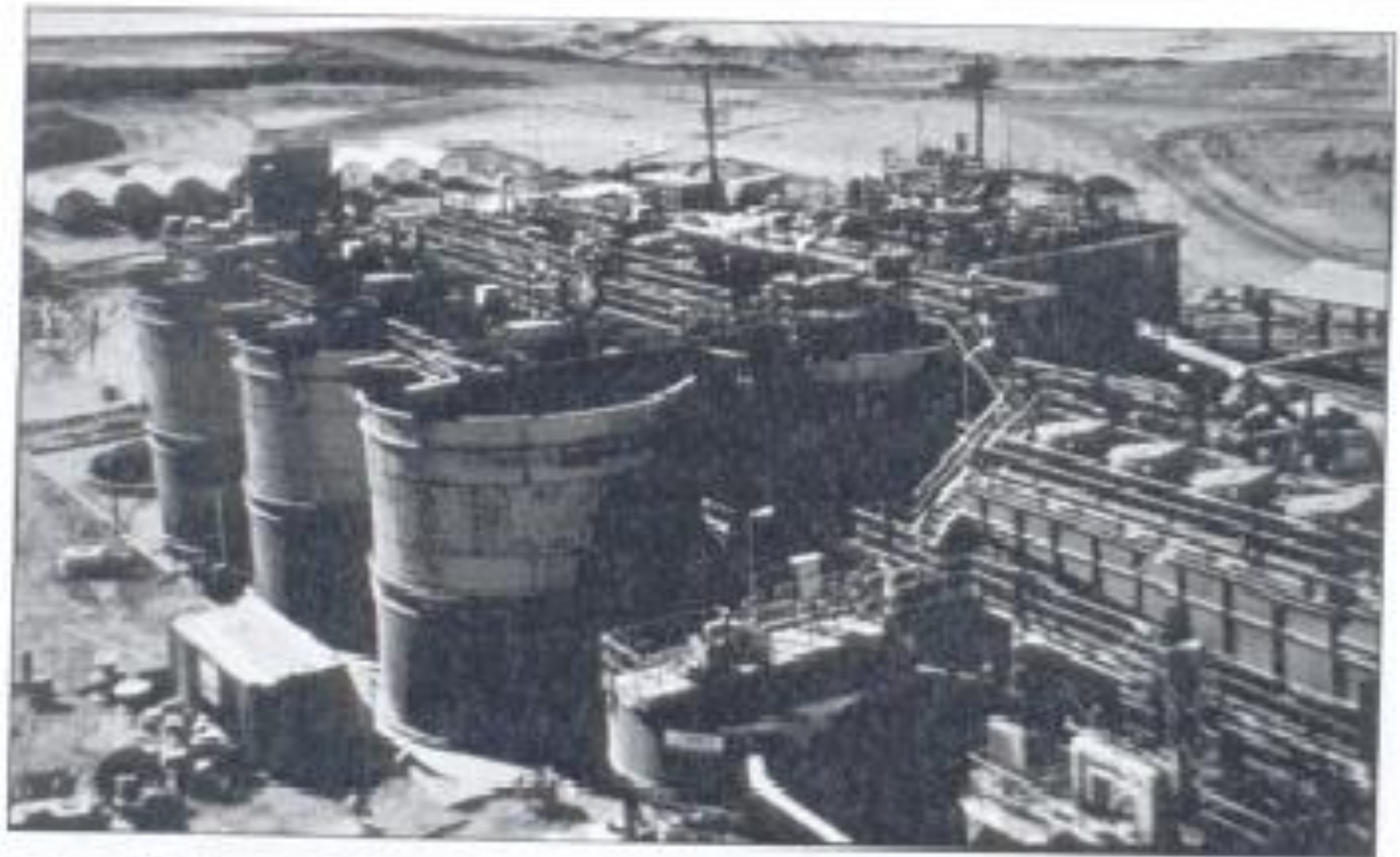
Fig. 1.1. At Youanmi Mine, Western Australia, 120 mt/day of refractory-sulfidic gold concentrate are biooxidized by moderately-thermophilic bacteria to enhance gold recovery.
